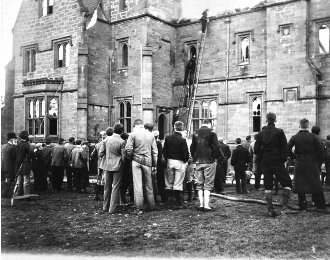
The morning after the fire at Trinity College Glenalmond 1894. Photo by A S Reid.
